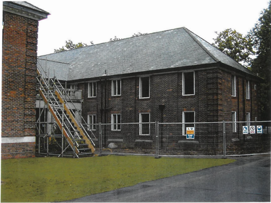
REAR VIEW SHOWING THE TEMPORARY EMERGENCY STAIRS
