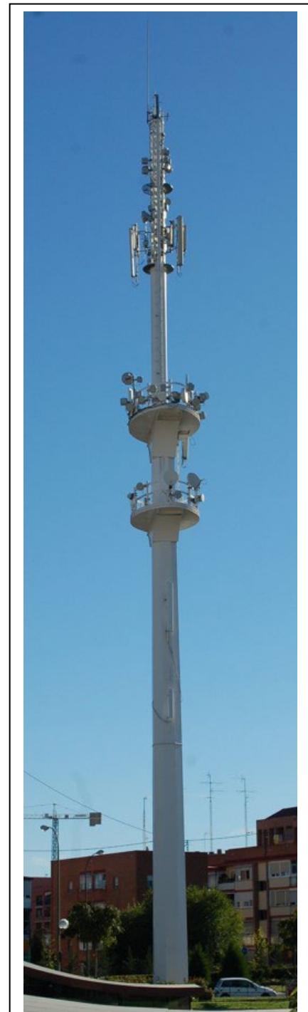
Utility Fixed Link radio Tower
