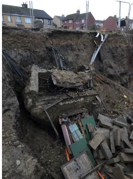
Figure 3.2: FTTC Cabinet for repair following landslip
